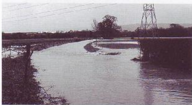
This is a road! – not a river
