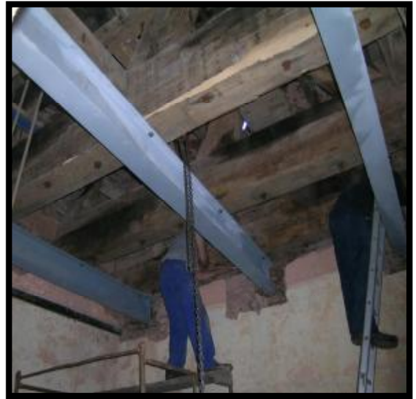
The new RSJ beams supporting the old timber bell frame support beams.
